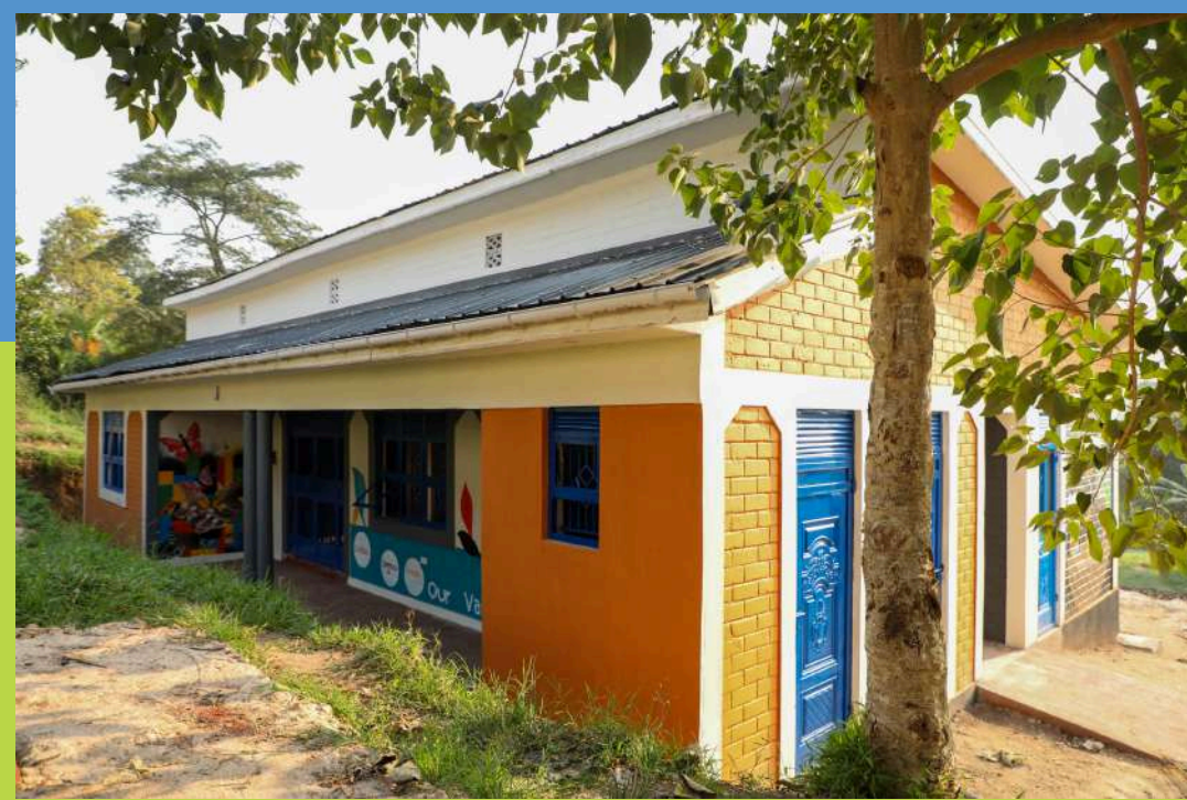
Completion of new multi-purpose building in the Rwamwanja Refugee Settlement at YINNOH
